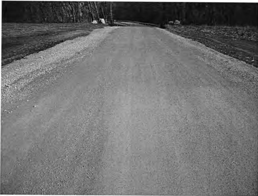
Figure 193. Control Section One on March 23, 2004
