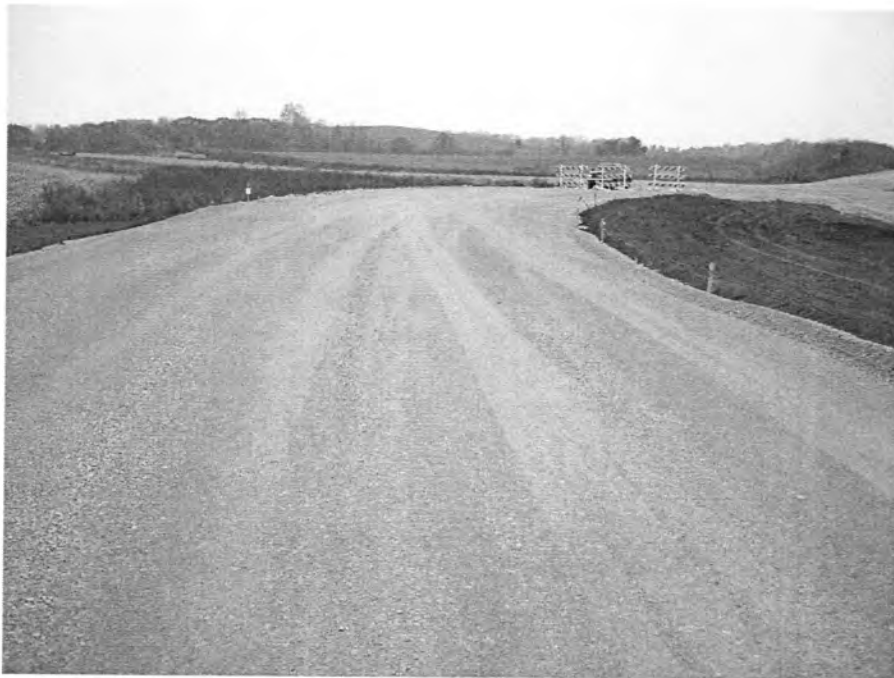
Figure 76. Completed Test Sections with Crushed Limestone Wearing Surface
