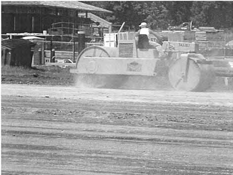
Figure 7. Final Compaction Using a Flat Drum Roller
