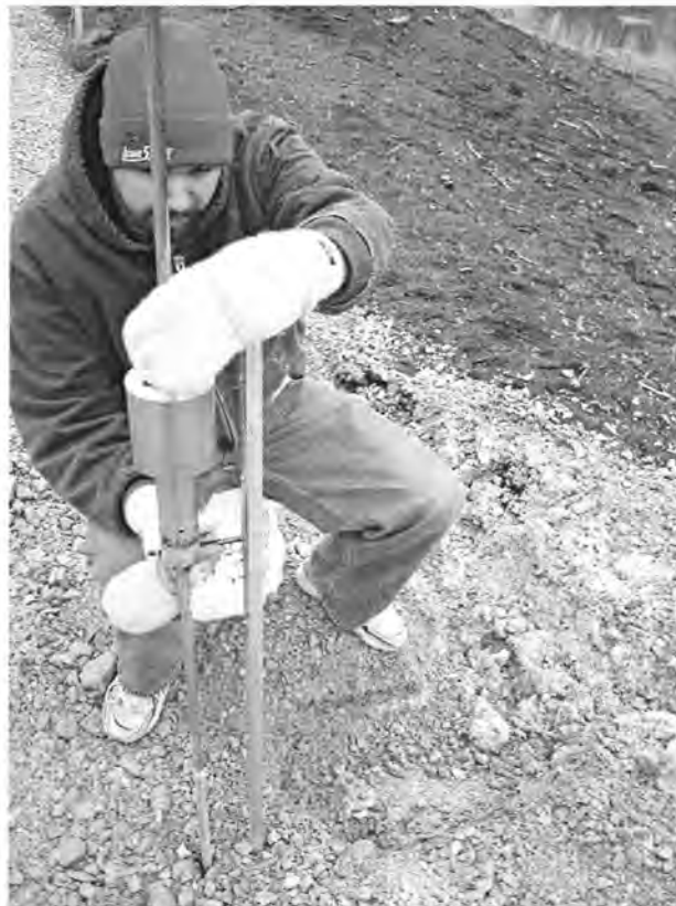
Figure 200. DCP Testing on March 2, 2004
