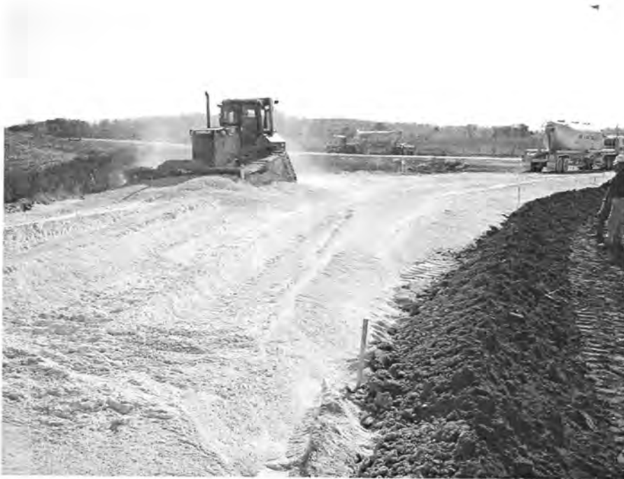
Figure 70. Spreading CKD in Test Section One
