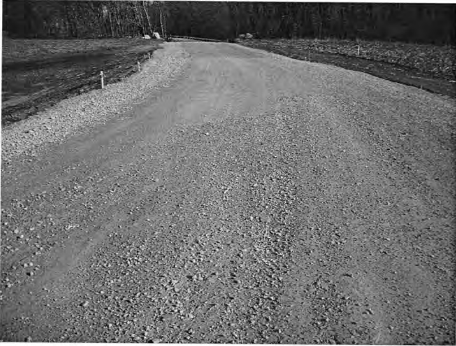
Figure 192. Test Section Two on March 23, 2004
