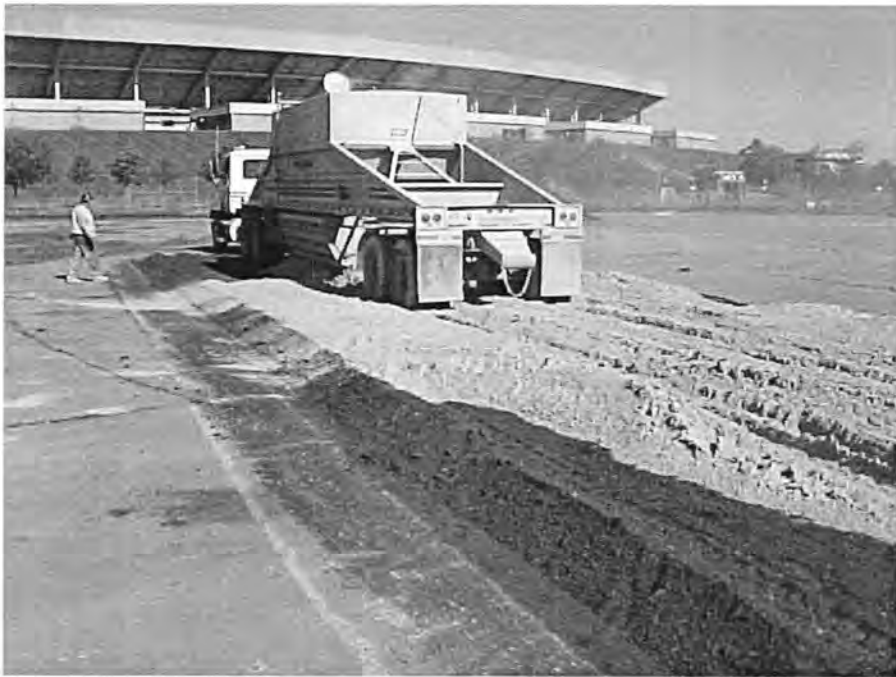
Figure 4. Addition of Class C Fly Ash from Bottom Dump
