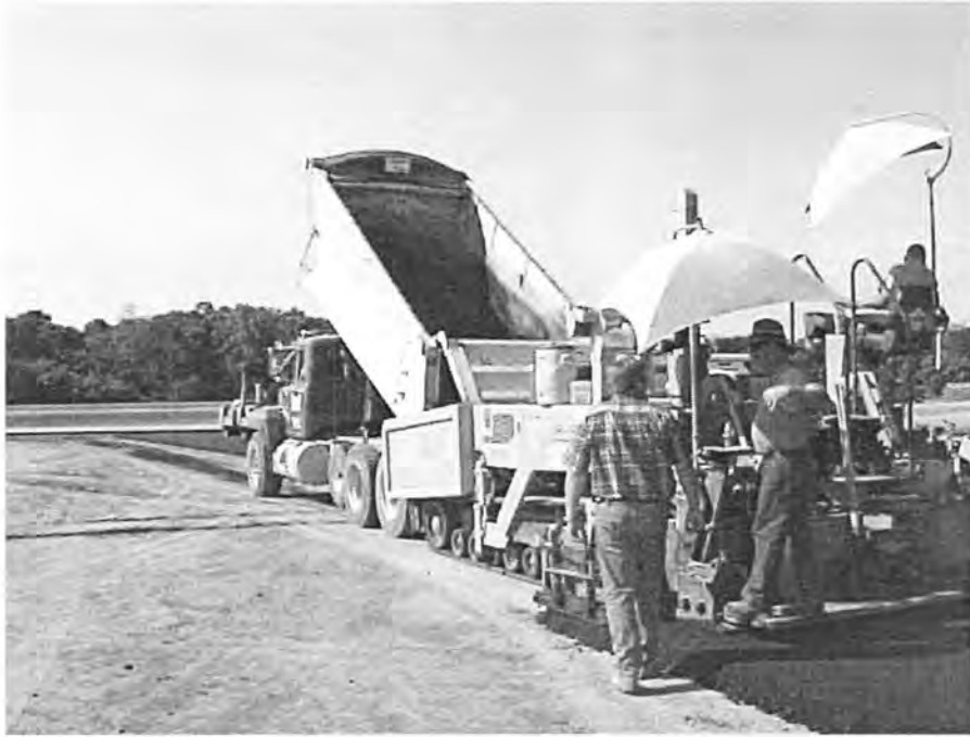
Figure 9. Placement of the Hot Mix Asphalt Surface
