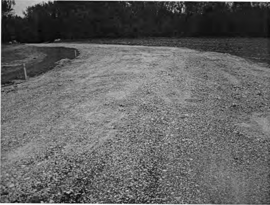
Figure 195. Test Section One on April 30, 2004
