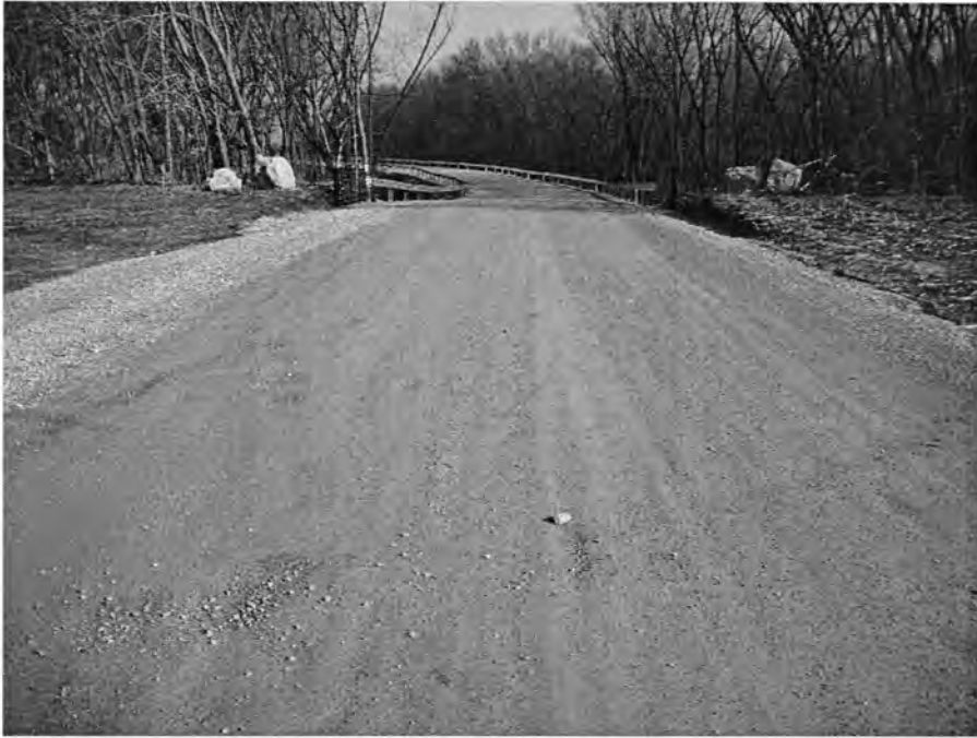
Figure 194. Control Section Two on March 23, 2004
