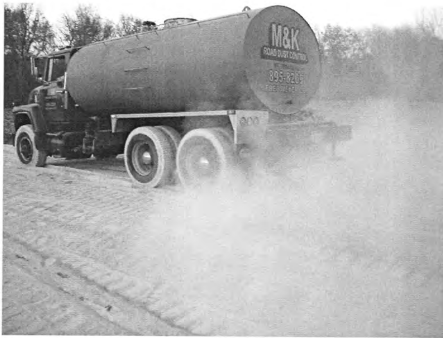
Figure 75. Watering of Stabilized Sections to Ensure Proper Hydration
