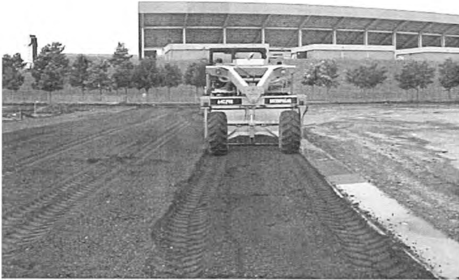
Figure 2. Milling of Existing Asphalt Surface
