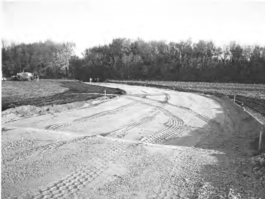
Figure 65. Test Sections One and Two before Placement of Limestone Screenings
