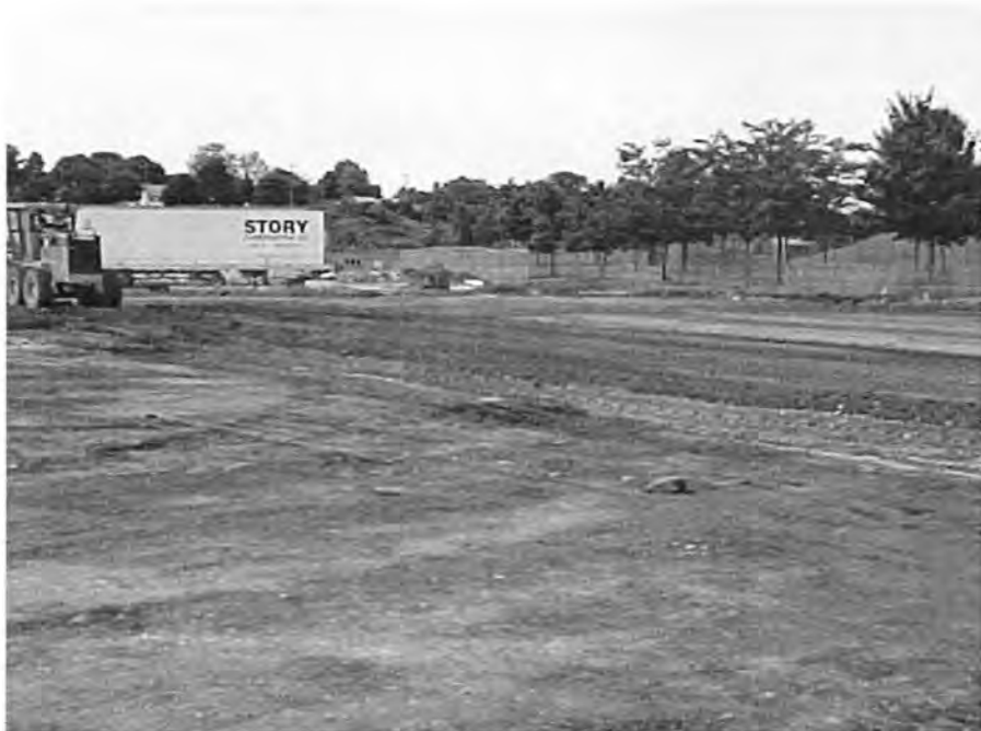
Figure 8. Final Grading with Motor Grader
