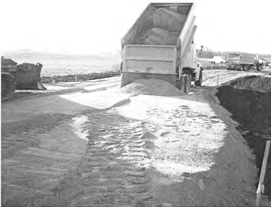
Figure 66. Placement of Limestone Screenings
