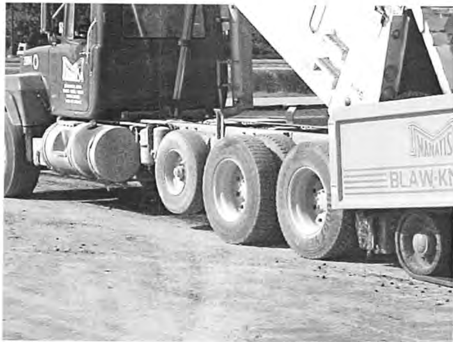
Figure 18. New Paving Platform without Rutting
