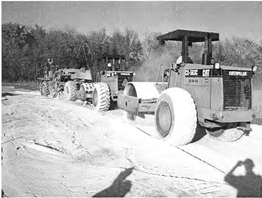
Figure 74. Mixing, Initial, and Final Compaction in Test Section Two
