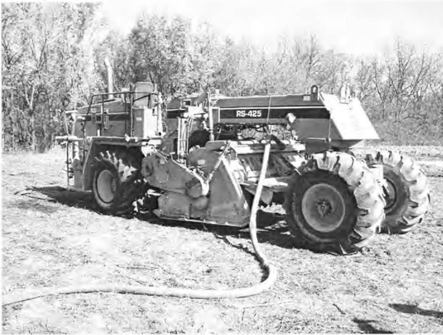
Figure 71. CMI RS 425 Road Reclaimer Used for Mixing
