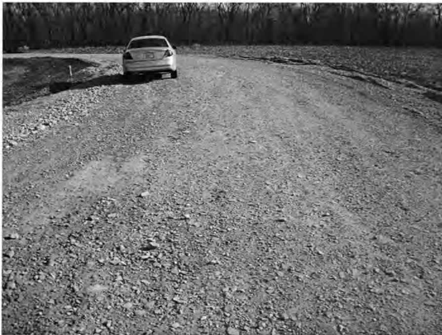
Figure 191. Test Section One on March 23, 2004
