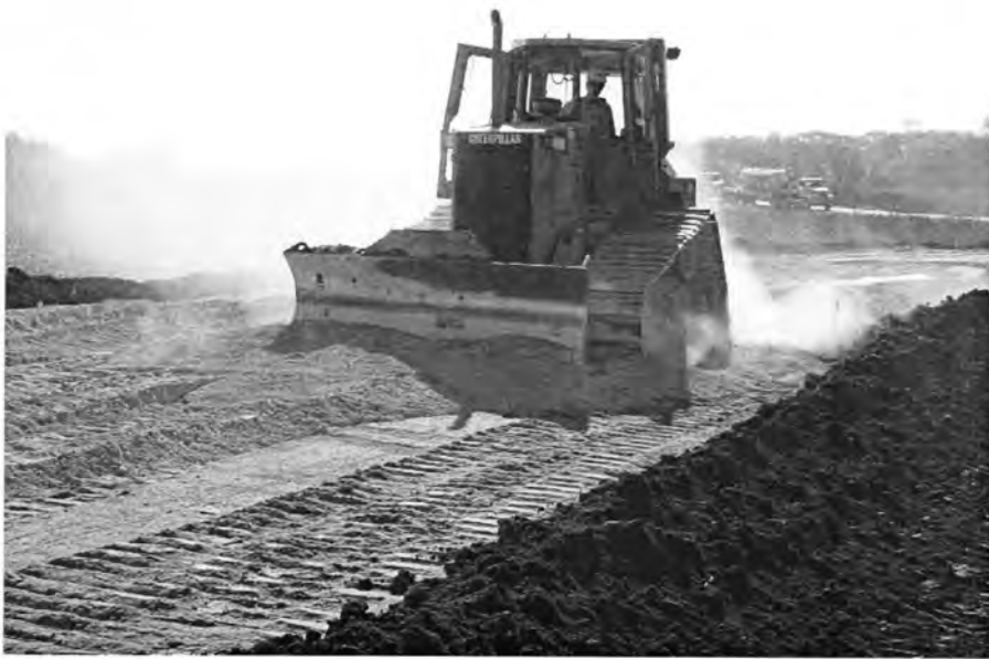
Figure 68. Spreading of Fly Ash with a Bulldozer
