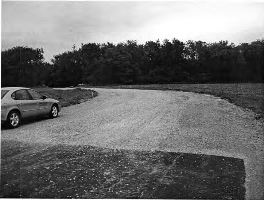
Figure 198. Test Section One on May 21, 2004
