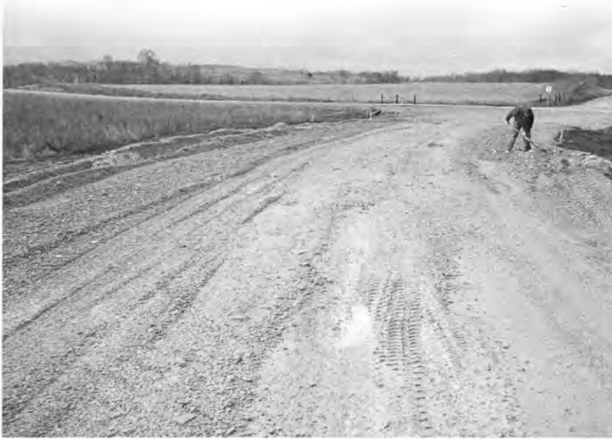
Figure 189. Failed Test Section One March 2, 2004 with Macadam Stone and Rutting
