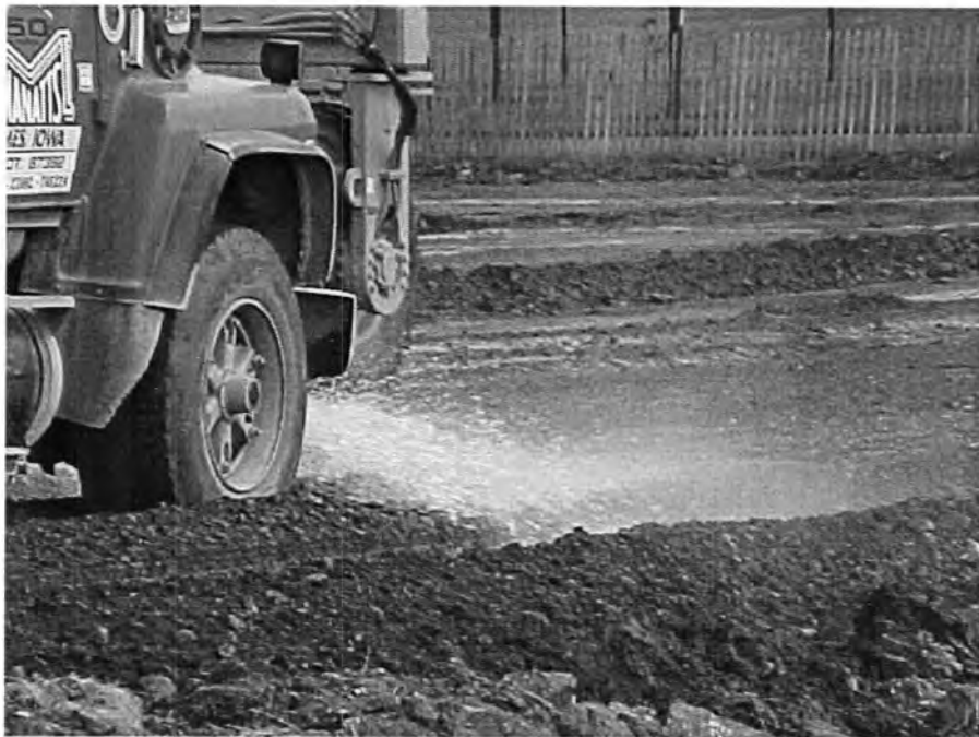
Figure 3. Addition of Water to Subgrade
