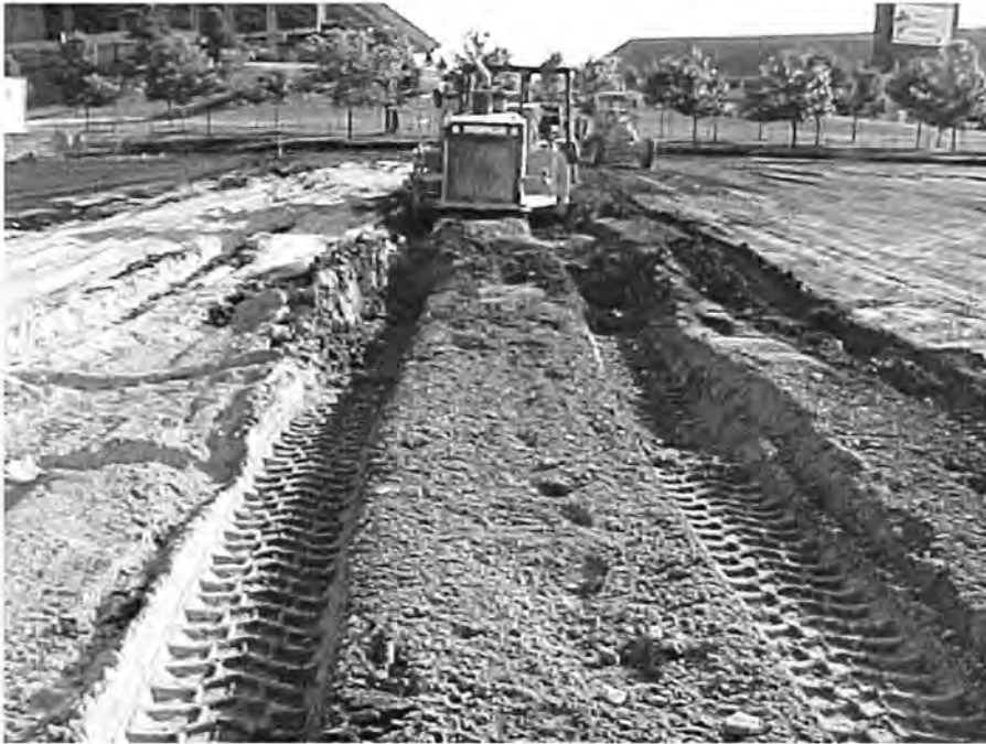
Figure 5. Mixing of Class C Fly Ash, RAP, and Subgrade Soil
