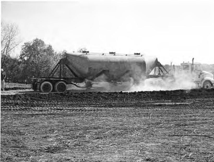
Figure 69. Placement of CKD in Test Section One and Two
