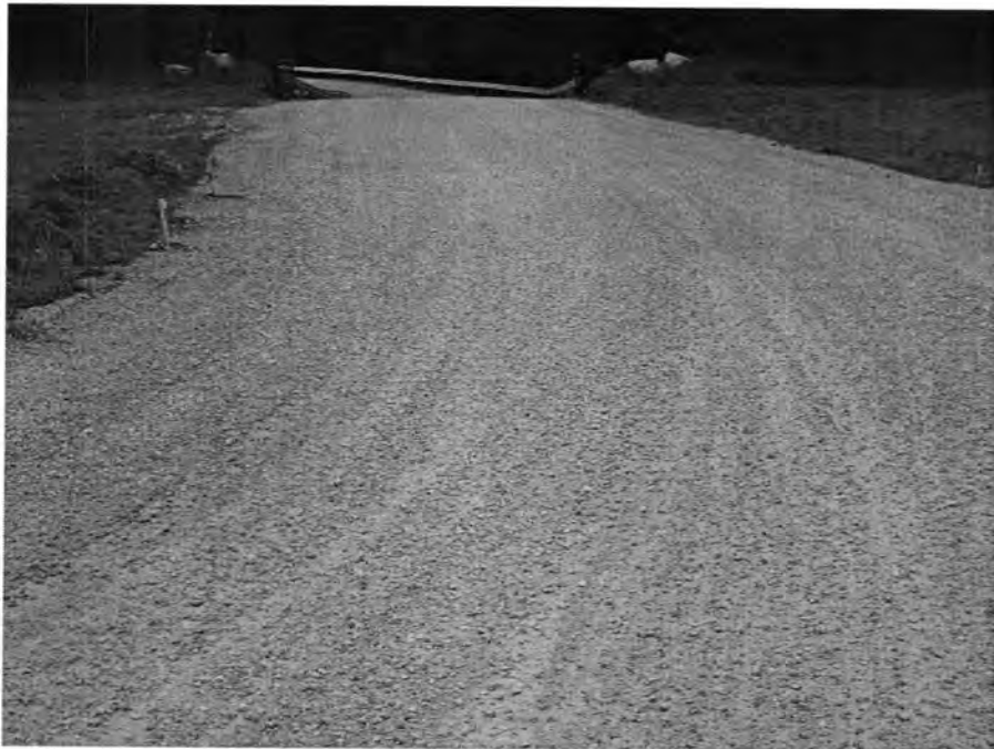
Figure 199. Test Section Two (Foreground) and Control Section One (Background) on May 21, 2004
