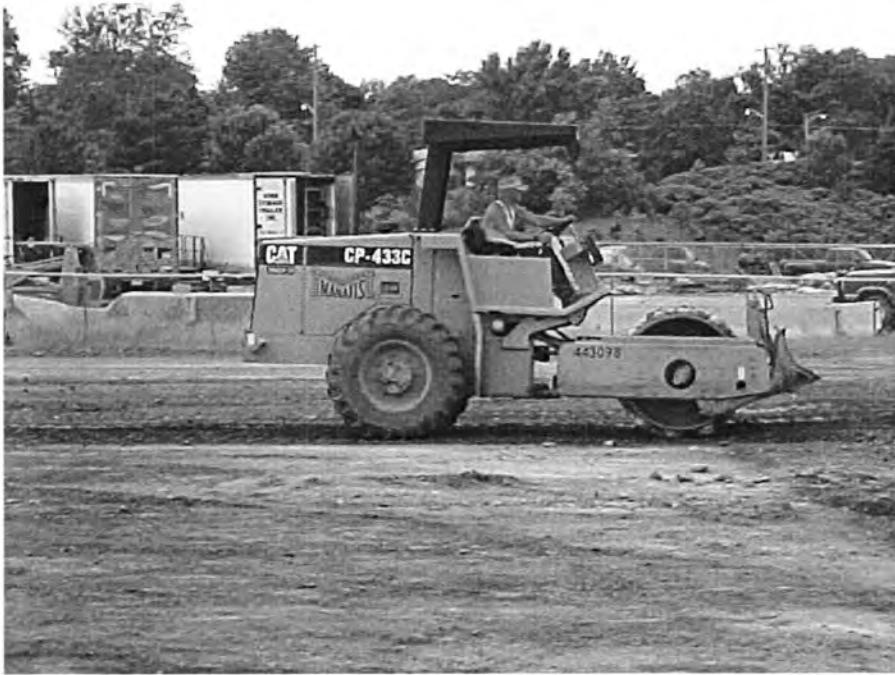
Figure 6. Initial Compaction Using a Vibratory Padfoot Roller
